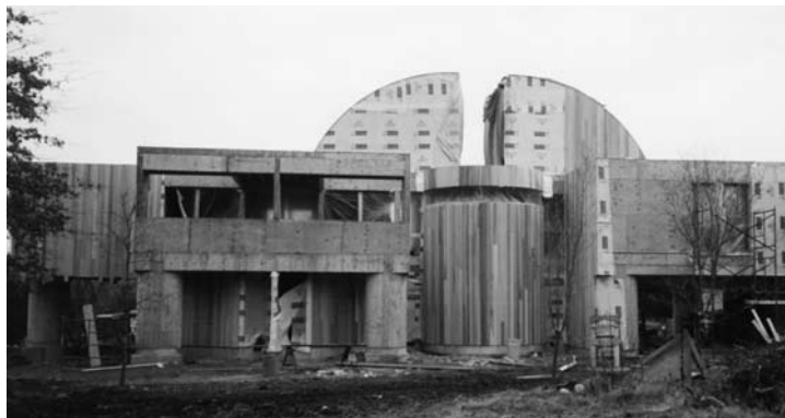
Errera Residence, Woodbridge, CT., during cedar siding installation.
