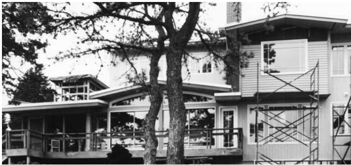
Sella Residence, Branford, CT., during construction.
