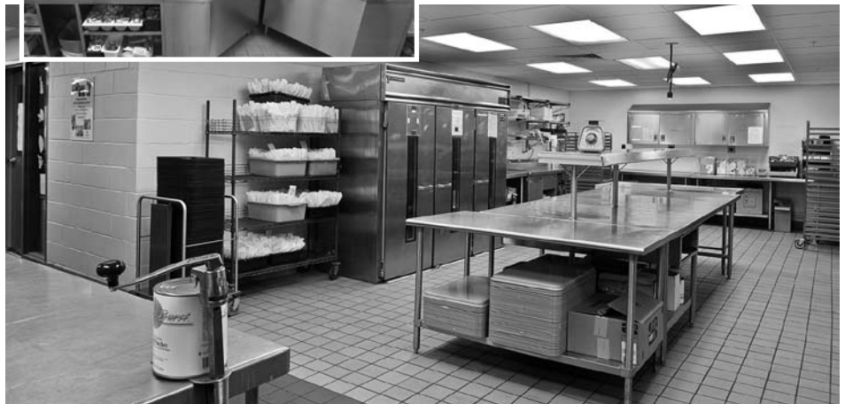
The newly renovated kitchen at Yale-New Haven Hospital is ready for service
